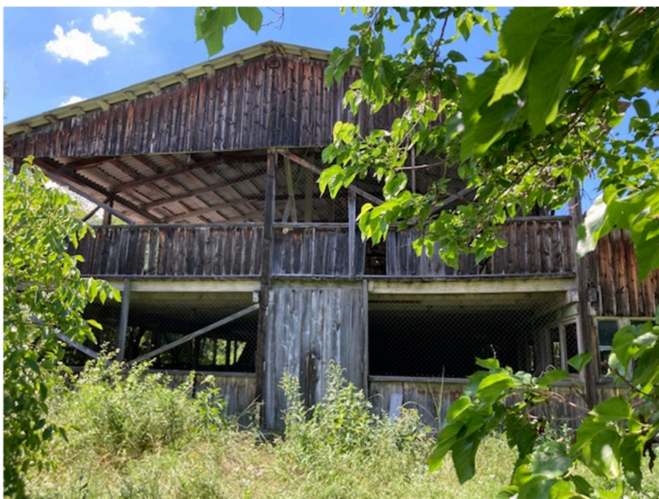
A Soviet era cocoon collection & drying facility in Akhmeta municipality
